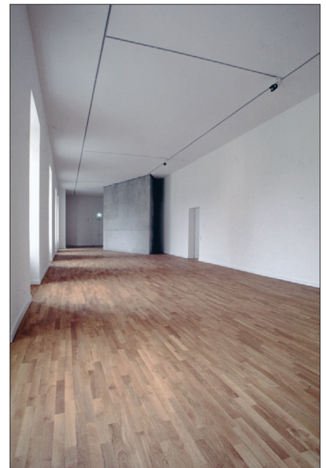
Oak parquet flooring impregnated with IRSA Natura Hard Oil in the Jewish Museum in Berlin
