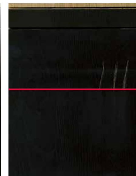
repaired (under the red line)
